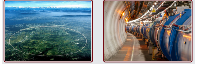
Fig. 1. The 27 km LHC tunnel, housing the LHC accelerator, here showing the superconducting magnets containing the two beam pipes. [27].
